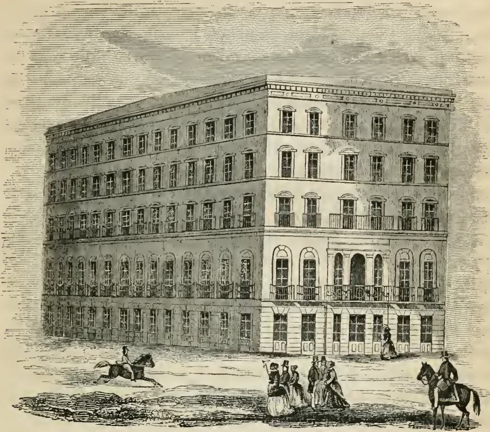
New Rasette House.
